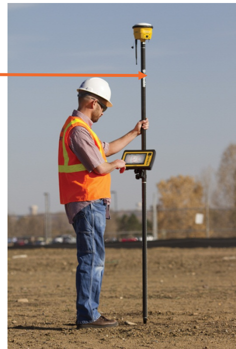
Rover Moves about the jobsite
