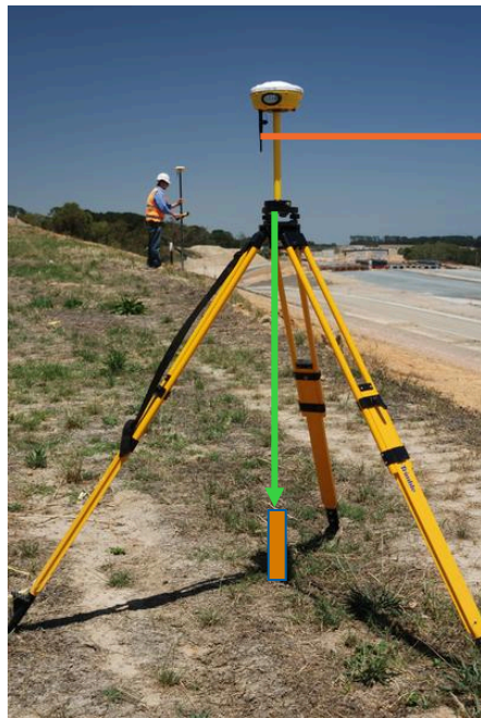
Base Station Set up over a fixed known point
